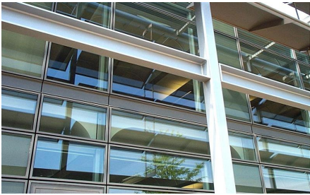
Wessex Water Operations Centre, Bennetts Associates
